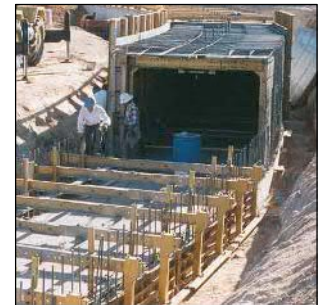
TYPICAL IMAGE OF INSITU CONCRETE PORTAL CULVERT
