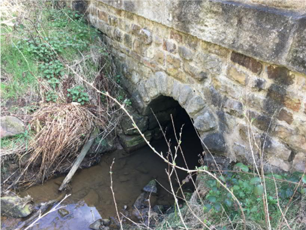
Figure 2 – Photo showing typical elevation on existing Structure B
