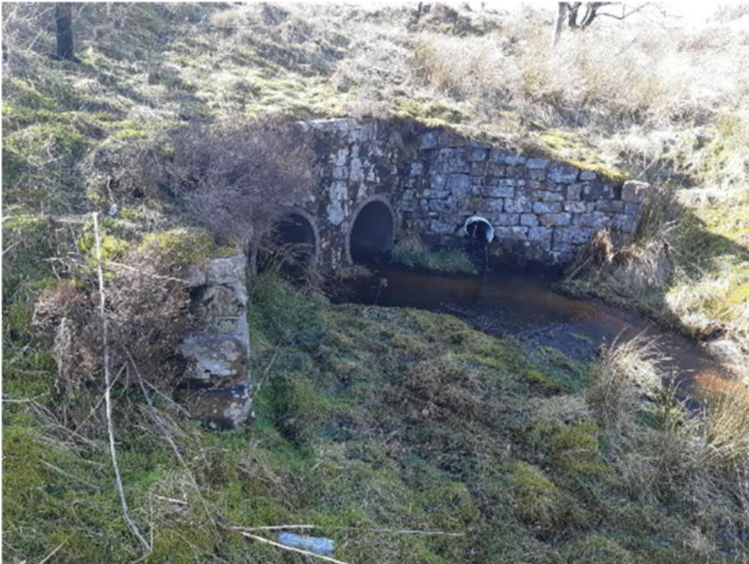
Figure 1 – Photo showing eastern headwall of existing Structure A
