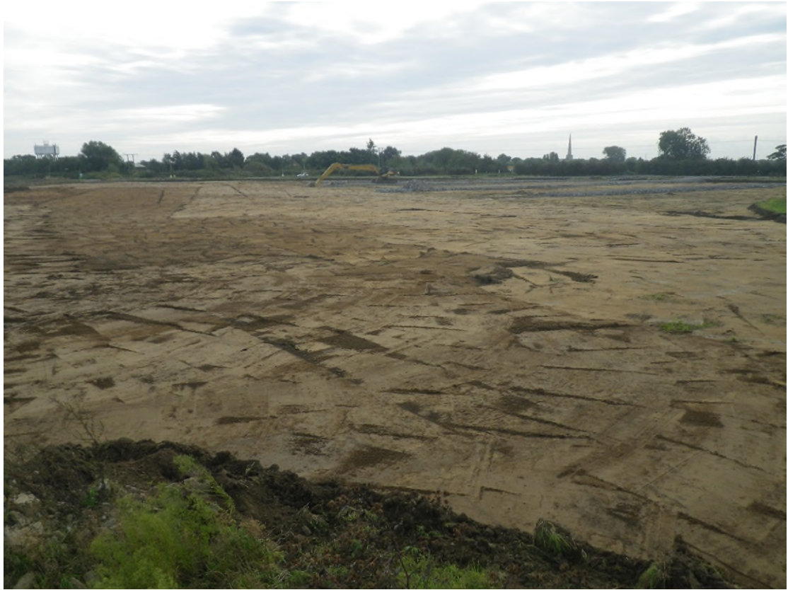
Plate 13 – Overall view of site following topsoil stripping, looking east
