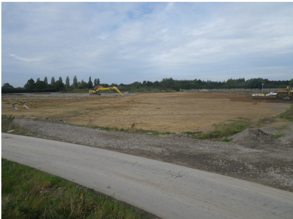
Plate 12 – Overall view of site following topsoil stripping, looking west
